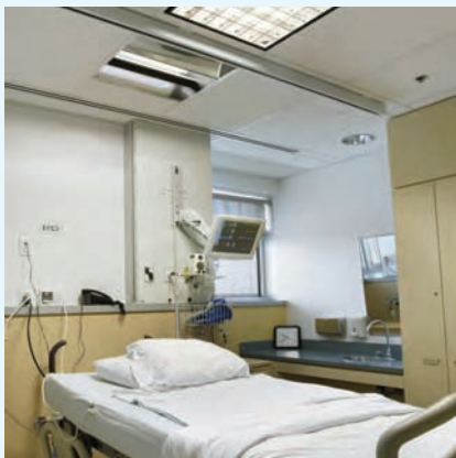
Luminaires featuring Lightolier, Vista and Alko
